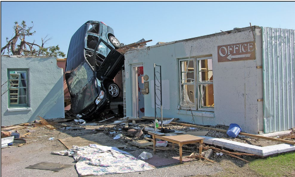
Figure B3-13. Vehicle rollover hazard (Greensburg, KS, 2007 tornado)
